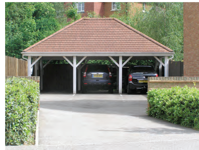
Example of well integrated car parking fronting onto a public space, including an example of a flat over garage (top).
