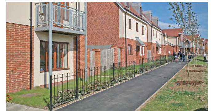
An example of a typical garden depth with railings that clearly define private space from public space.
